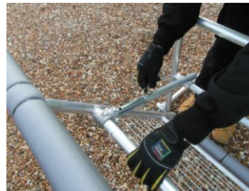
Fig 3. Lowering the panel frame
