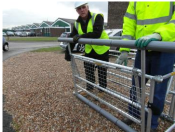
Fig 3. Lowering the panel frame
