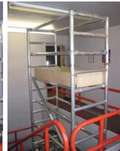
11. Climb partially onto this platform through the trapdoor and adopt the 3T position as described earlier and then fit four 1.5m horizontal guard rail braces at 0.5m and 1.0m above the platform as shown.
