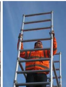
9. Now climb fully onto this platform and close the trapdoor behind you. Fit the four rung guard rail frame to the top of the frames on the upper step and the three rung guard rail frame to the top of the frames on the lower step. Lock the interlock clips to secure the frames together.
